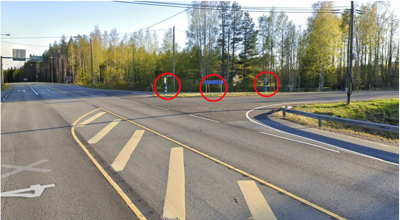
Pic 39/pos 20. Road 4 in Elämäjärvi. Turning right and removing traffic signs. PHOTO FAILED, USED GOOGLE MAPS STREET VIEW IMAGE
