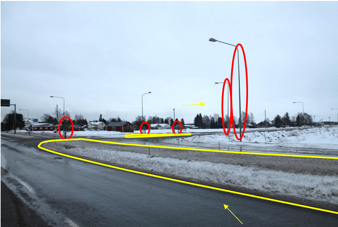
Pic 13/pos 4. Turning from road 8 toward road 27. Marked lamp posts and signs need to be removed. Marked areas need to be filled. Yellow arrow points driving direction.
