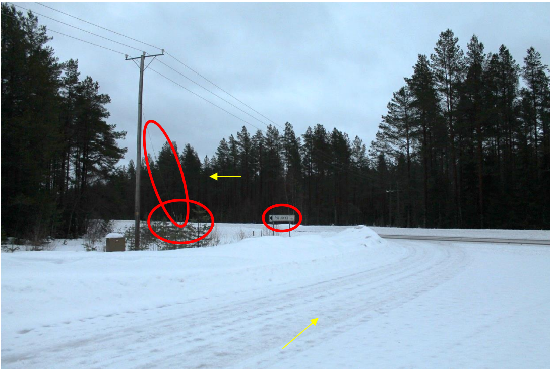
Pic 7/pos 1. Turning from Repolantie toward Satamatie (road 7771). Marked sign and wire need to be removed. Marked trees need to cut. Yellow arrow points driving direction.
