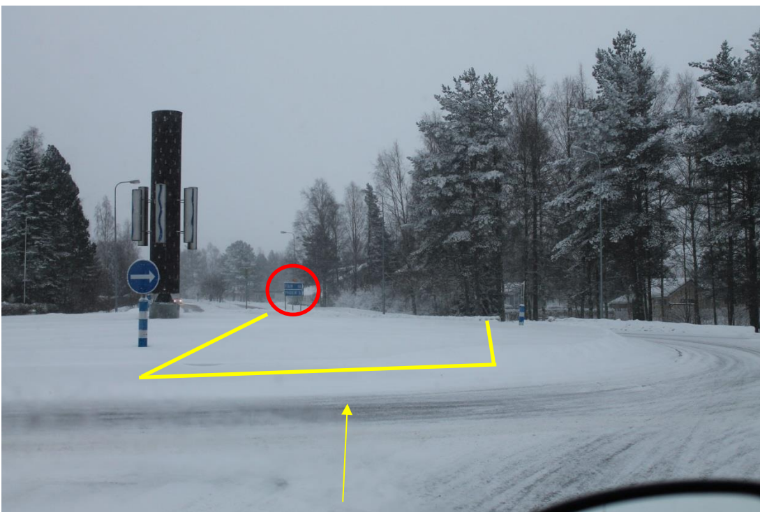
Pic 34/pos 18. Roundabout in Haapajärvi. Marked sign need to be removed. Marked area need to be filled. Yellow arrow points driving direction.
