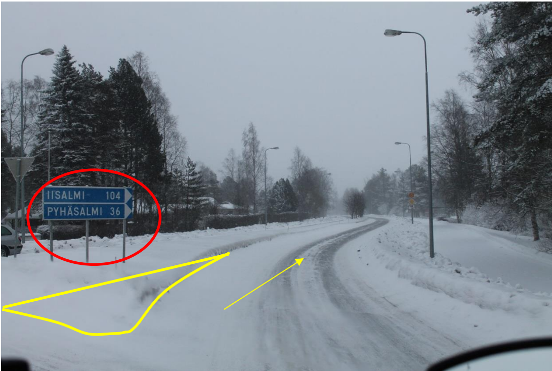
Pic 35/pos 18. Roundabout in Haapajärvi. Marked sign need to be removed. Marked area need to be filled. Yellow arrow points driving direction.
