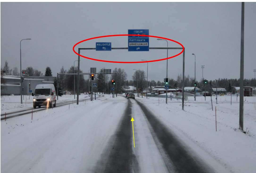
Pic 30/pos 16. Road 27 in Nivala. Marked portal need to be removed. Height 5,70m. Yellow arrow points driving direction.
