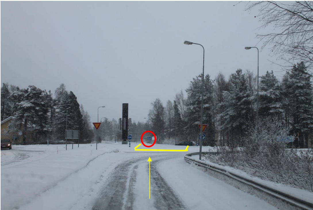
Pic 33/pos 18. Roundabout in Haapajärvi. Marked sign need to be removed. Marked area need to be filled. Yellow arrow points driving direction.
