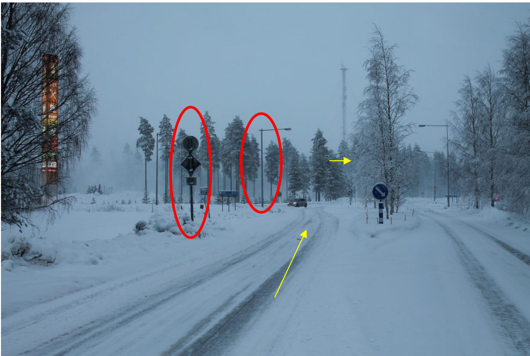
Pic 36/pos 19. Turning from road 27 toward road 4. Transports take counter lane. Marked lamp post and sign need to be removed. Yellow arrow points driving direction.
