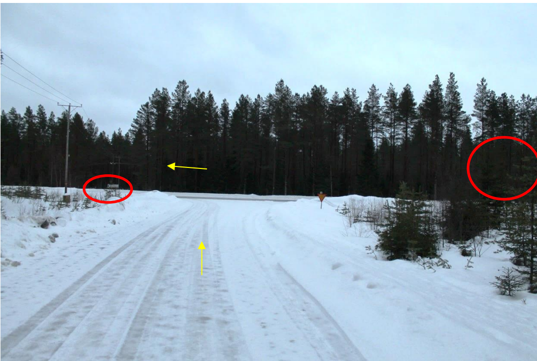
Pic 6/pos 1. Turning from Repolantie toward Satamatie (road 7771). Marked sign need to be removed. Marked trees need to cut. Yellow arrow points driving direction.
