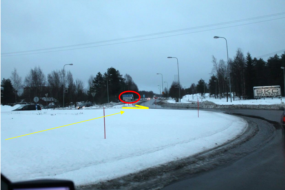
Pic 17/pos 7. First roundabout in Ylivieska. Marked sign need to be removed. Marked area need to be filled. Yellow arrow points driving direction.
