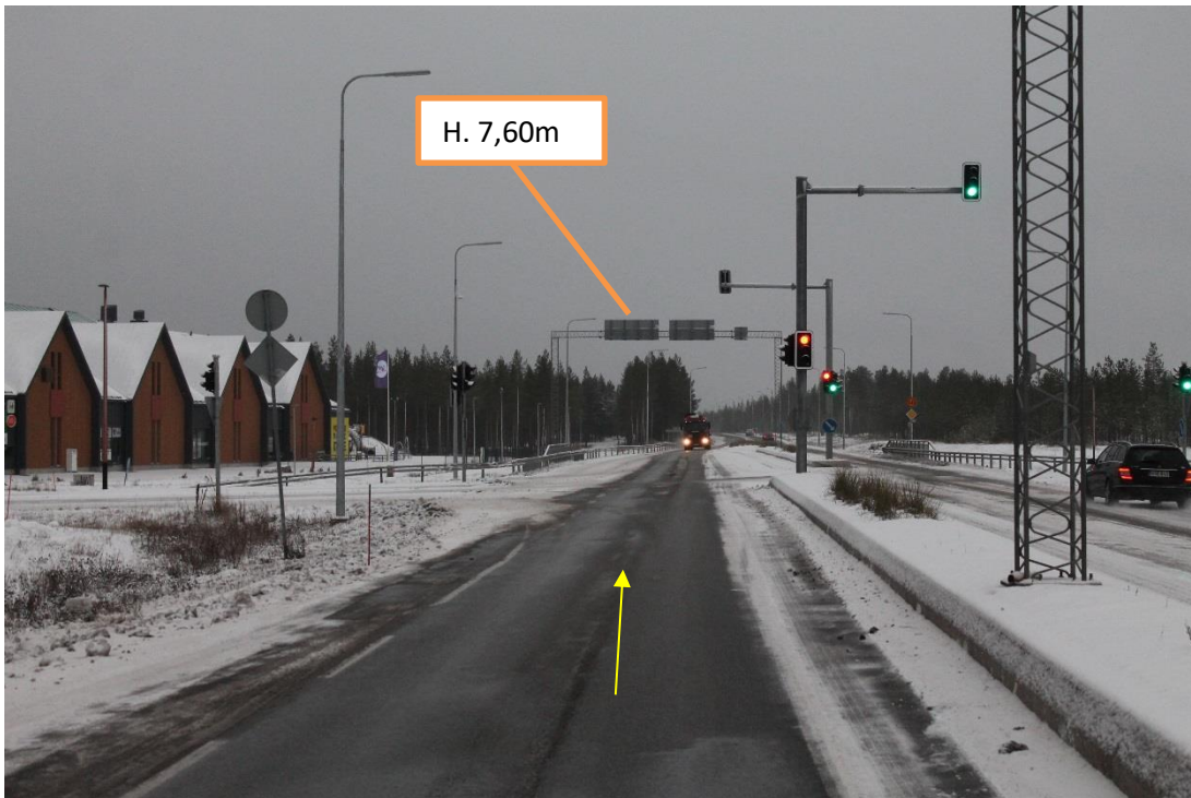
Pic 11/pos 3. Road 8. Transports continue on counter till end of traffic island. Height of the portal is 7,60m. Yellow arrow points driving direction.
