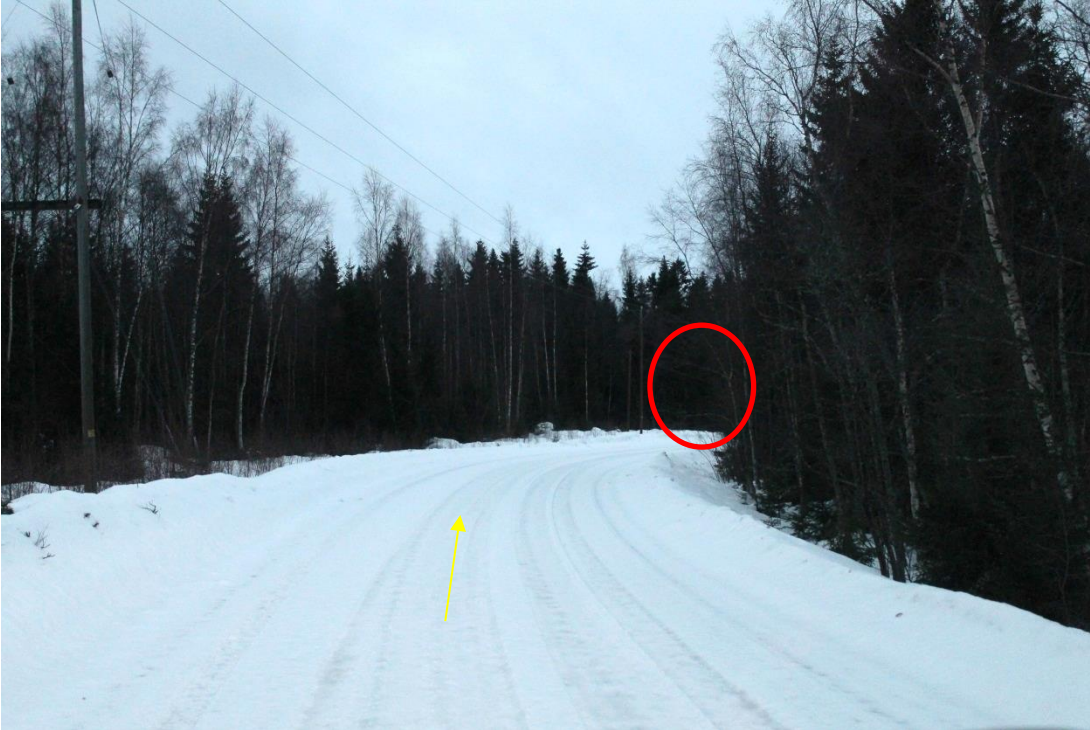
Pic 5/ pos A2. Repolantie. Some tree branches need to cut on the Repolantie. Yellow arrow points driving direction. Yellow arrow points driving direction.
