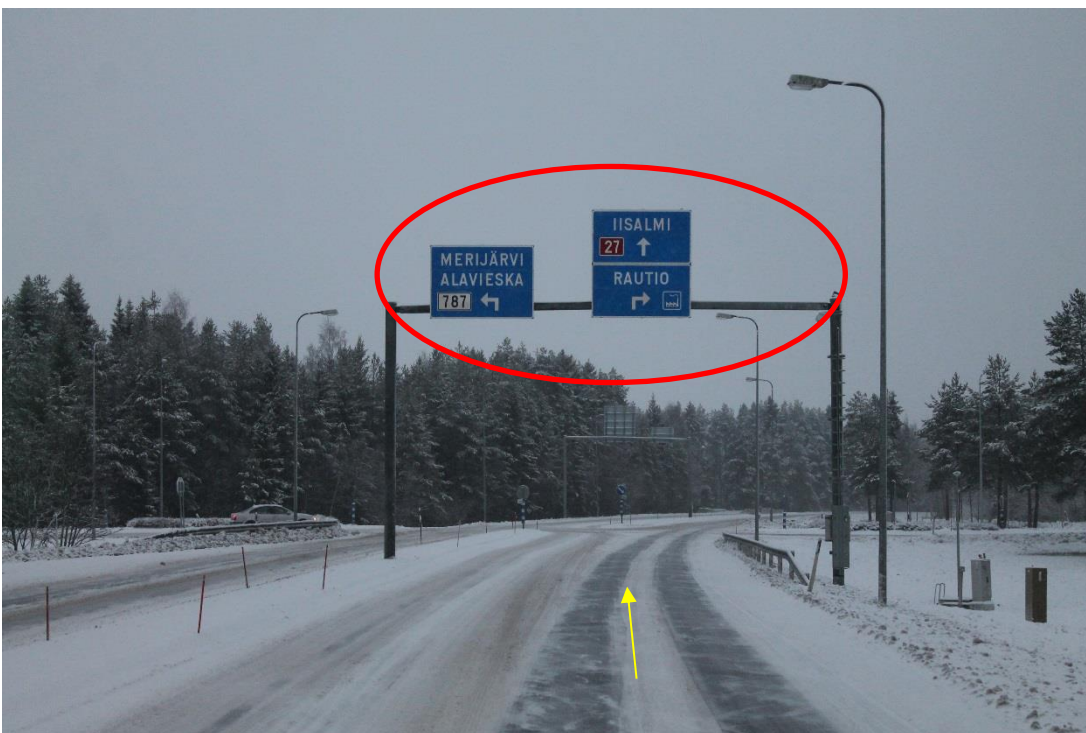
Pic 14/pos 5. Road 27. Marked portal need to be removed. Portal height 6,15m. Yellow arrow points driving direction.
