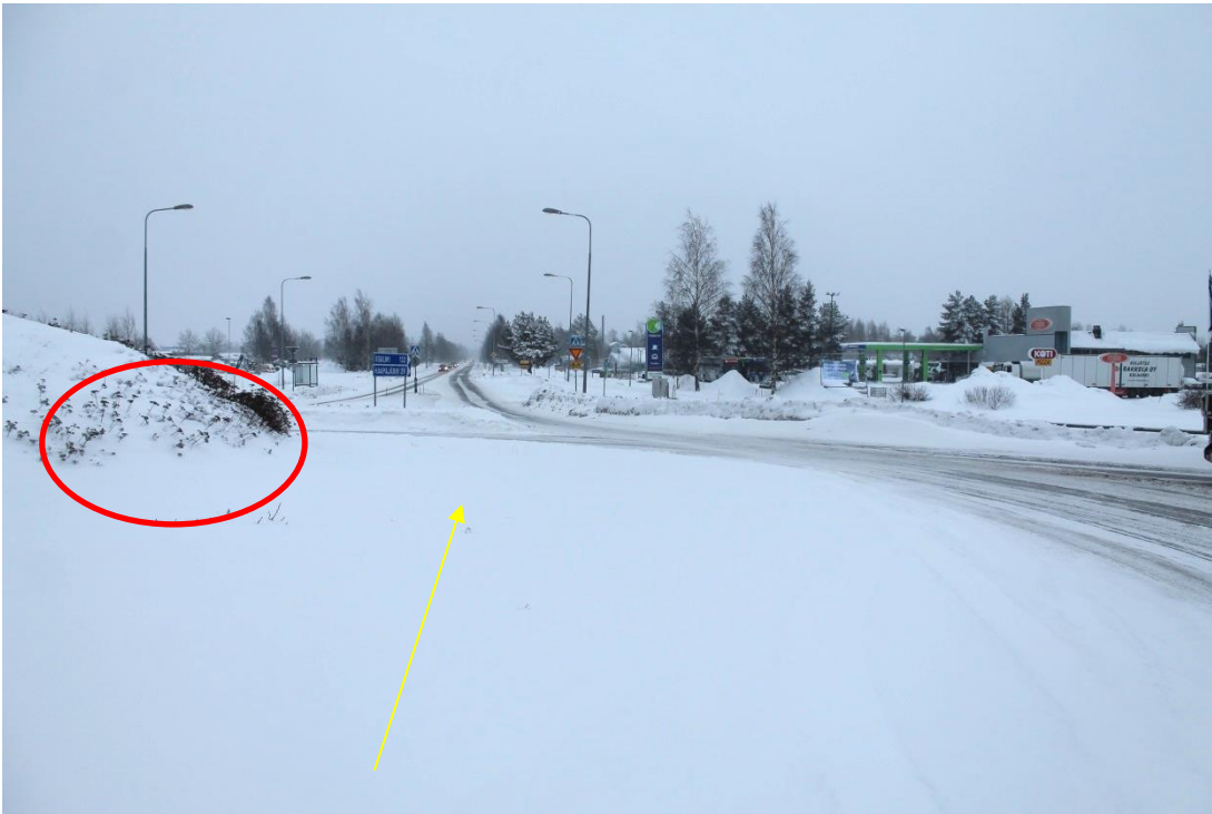
Pic 27/pos 14. Roundabout in Nivala. Marked area need to be flat. Yellow arrow points driving direction.
