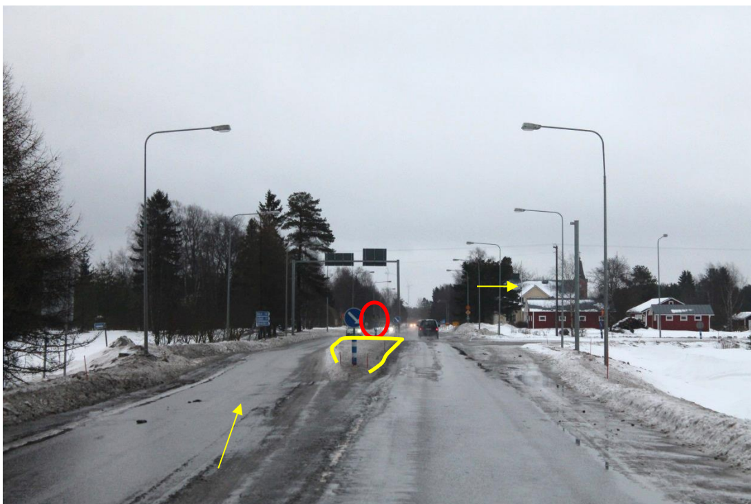
Pic 12/pos 4. Turning from road 8 toward road 27. Marked sign need to be removed. Marked area need to be filled. Yellow arrow points driving direction.
