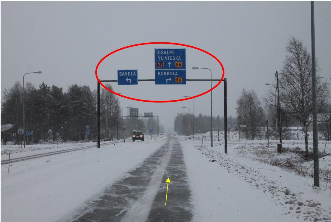
Pic 15/pos 6. Road 27. Marked sign need to be removed. Portal height 5,70m. Yellow arrow points driving direction.
