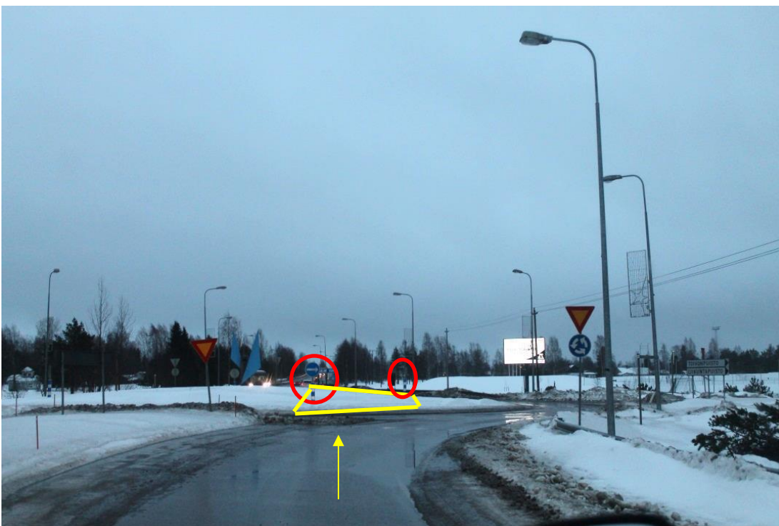
Pic 18/pos 8. Second roundabout in Ylivieska. Marked signs need to be removed. Marked area need to be filled. Yellow arrow points driving direction.
