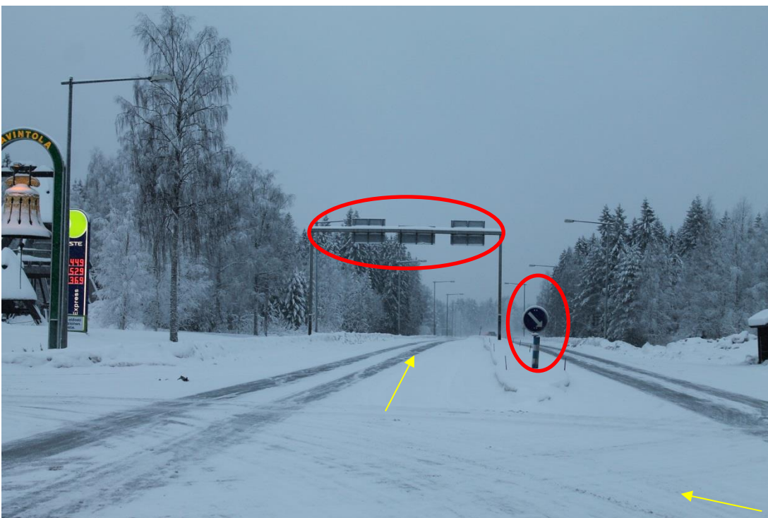
Pic 38/pos 19. Turning from road 27 toward road 4. Transports continue on counter lane till end of traffic island. Marked signs need to be removed. Yellow arrow points driving direction.
